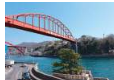
The Ondo Bridge spanning the "Ondo-no-Seto" (with Ondo in the foreground)
